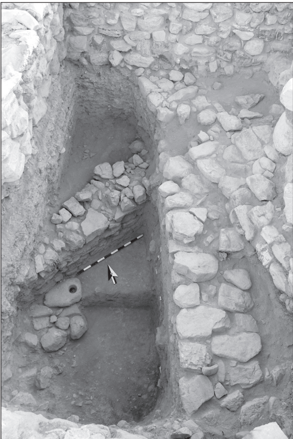
9. Area C, Square C6: EB III Subphase 1c stone wall and pivot stone with associated surface; looking north.
